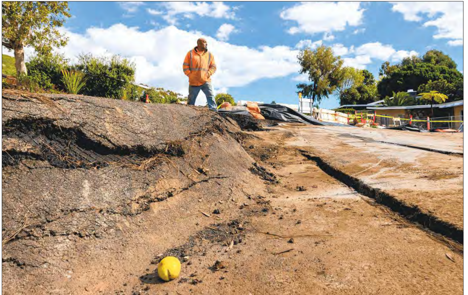
Photographs by BRIAN VAN DER BRUG Los Angeles Times
